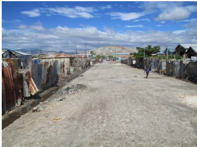
Figure 4 One of the paved streets in Jubilee
