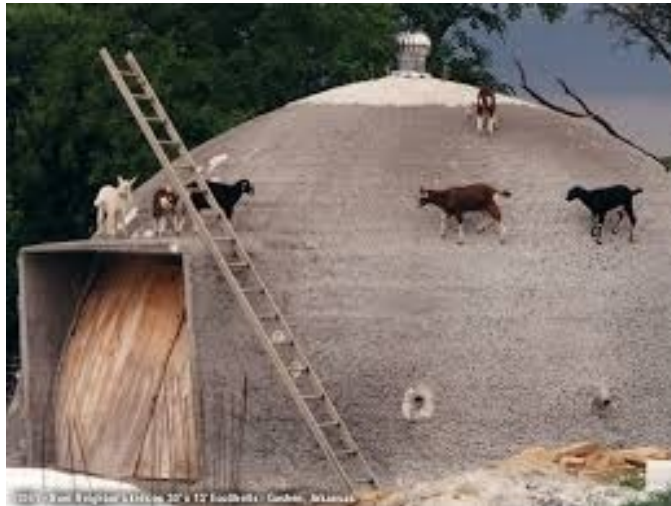
Figure 6 EcoShell I home under construction.
