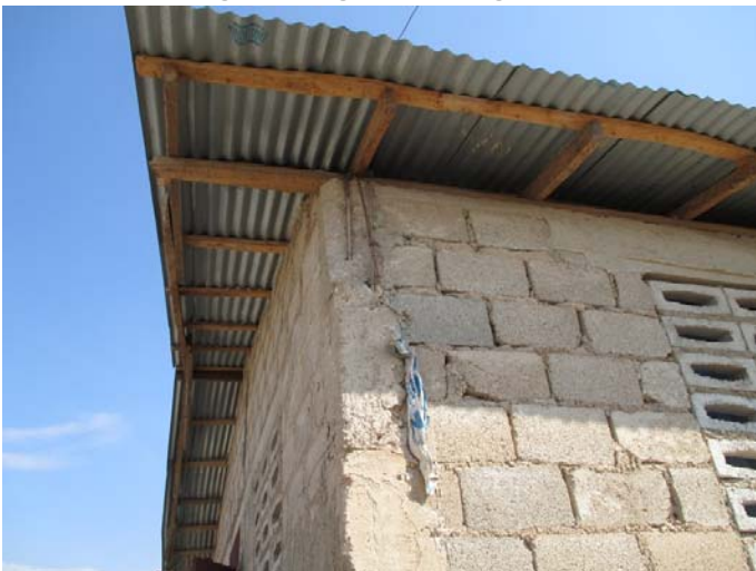
Figure 7 Confined Masonry Construction
