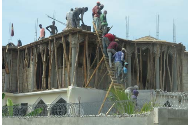
Figure 3. Pouring a roof on a 2nd story building.
