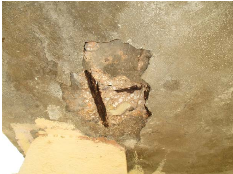
Figure 15. Bottom of overhead water tank.
