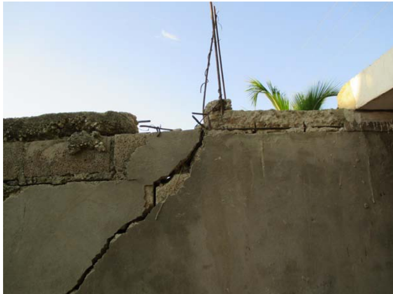
Figure 9. An inadequate foundation led to this wall cracking.
