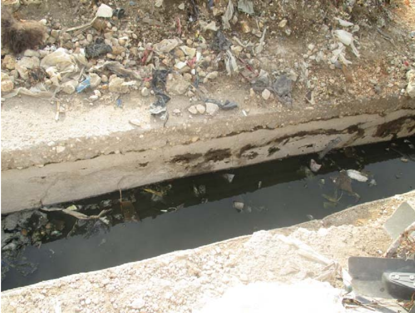
Figure 20. The new version of the open sewer.
