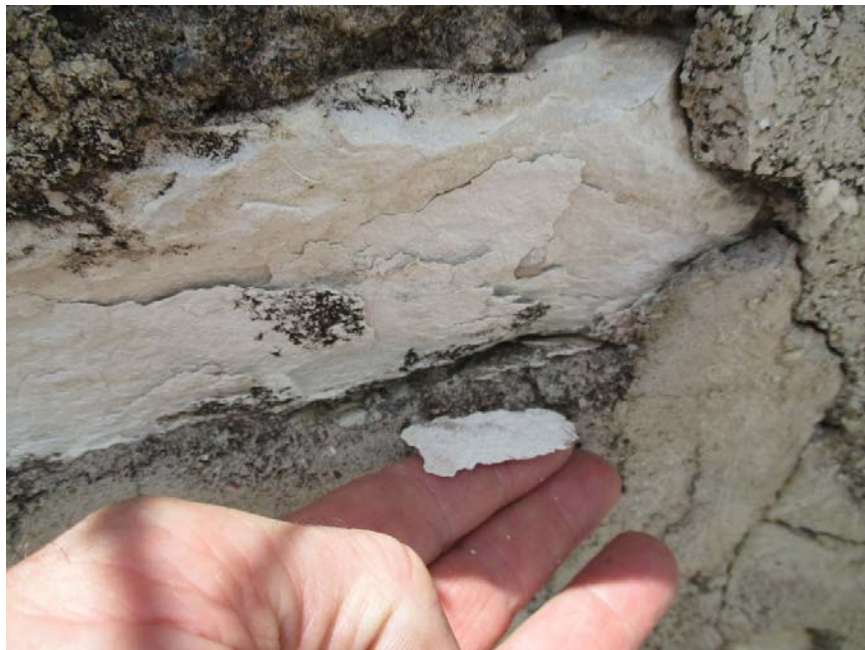
Figure 17. Deteriorating stone in sewer.
