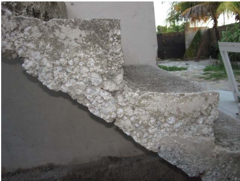
Figure 10. Porous concrete used to form an outside stair.
