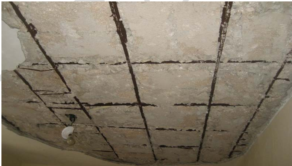
Figure 1. The underside of a “flat” concrete roof in Gonaives, Haiti
